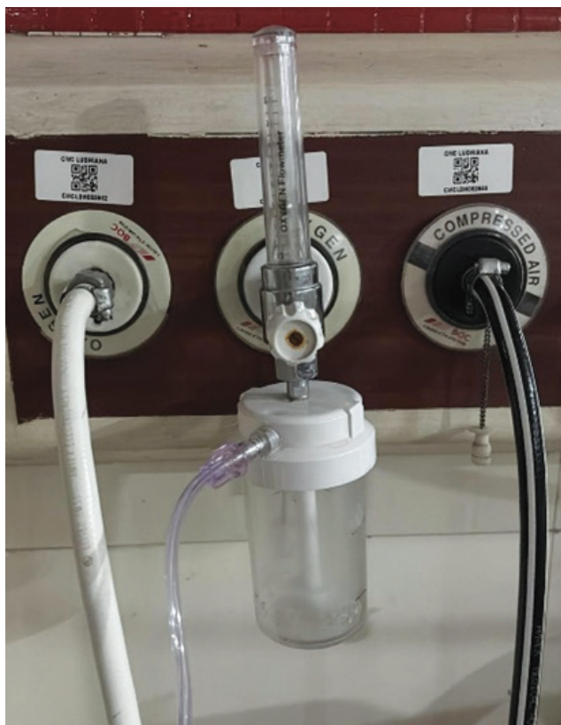
Fig. 2 Oxygen Flowmeter
